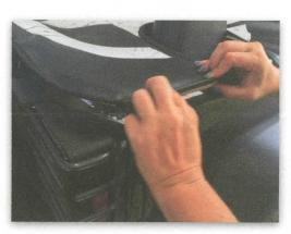
**Step 3:** Insert the white attachment channel tabs under the tub rails as shown. Start with the rear corner tabs then the sides. Insert one side, then move to the other.
