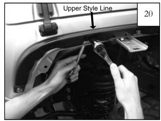
**Step 4** Using a 1/2" socket wrench and a 1/2" wrench, tighten all bolts until inner piece is snug against fender and washers do not spin. *NOTE: Do not overtighten:* See step 21. Inner piece should rest along upper style line of sheet metal radius and not below it: See step 22.
