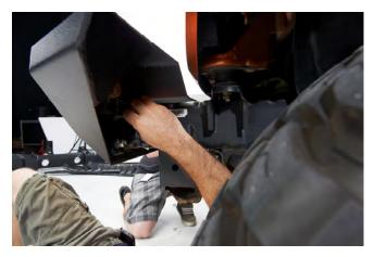
**STEP 6** // Slide the bumper in place. Using the supplied washers and nuts, secure the bumper to the frame.
