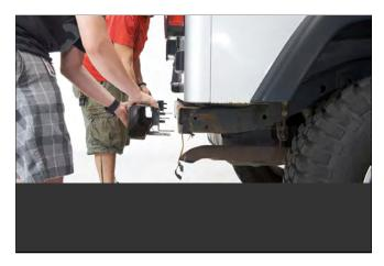
**STEP 4** // Slide the bumper away from the back of the vehicle.
